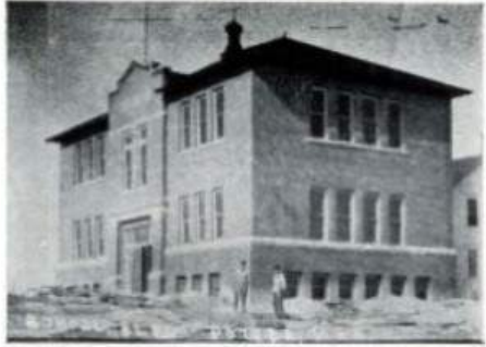
NEW $12,000 SCHOOL BUILDING, POTTER, NEB.
