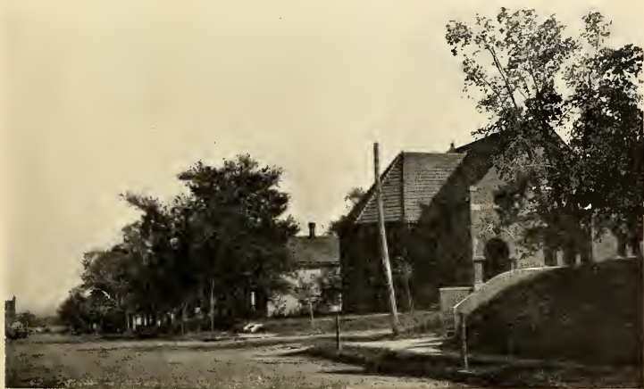
LIBRARY AND VIEW OF FIRST CORSO LOOKING EAST FROM TENTH STREET
