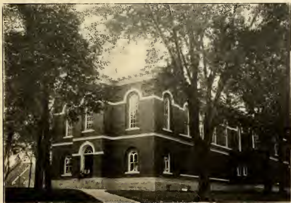
OTOE COUNTY COURT HOUSE
