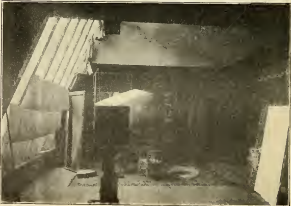
OPERATING ROOM OF PEASLEY
