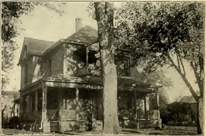
RESIDENCE OF MR. CHAS. McNAMARA
