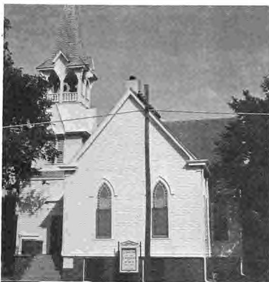
Remodeled Covenant Church
