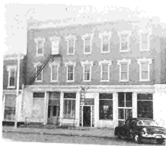
THE VIKING CENTER BEFORE CONSTRUCTION
