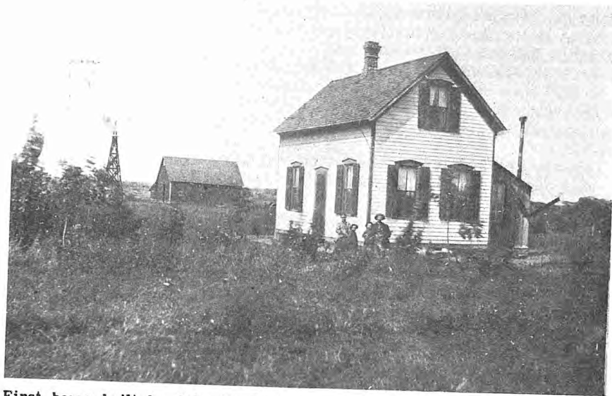
First home built by John F. Anderson on his homestead in the fall of 1878. In the picture are Mr. and Mrs. John F. Anderson and their sons, Ansel Edward and Fred Albin.
