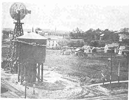
Windmill and water tower used for the big steam engines
