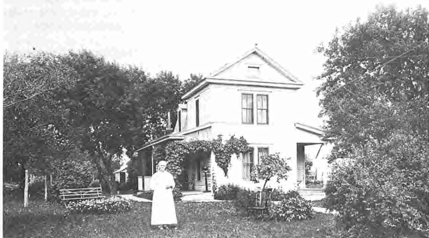
First home of Mr. and Mrs. P. O. Nordlund (after addition)
