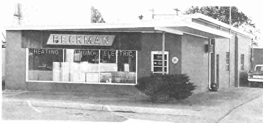
Beckman Plumbing Cooling Heating and Electric
