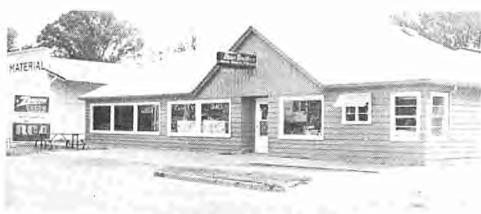
The present Moore Lumber Co. building
