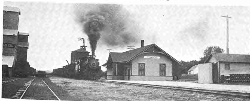
The Stromsburg depot
