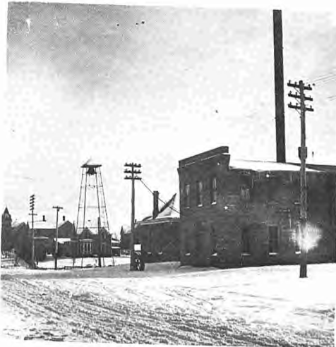
Electric light plant and fire bell.
